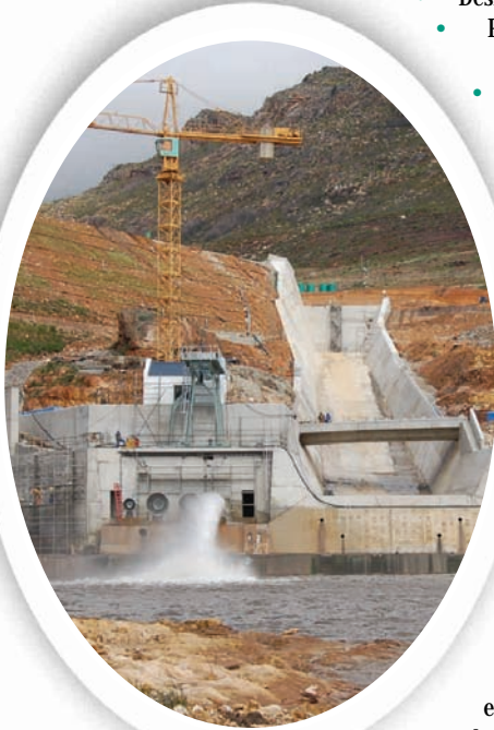
The Berg River Dam spillway and outlet works.
